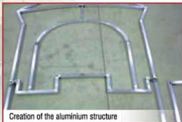
Creation of the aluminium structure
