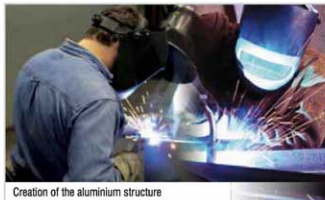
Creation of the aluminium structure
